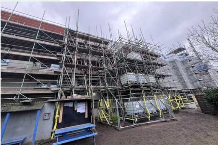
Phase 2 scaffolding ongoing
